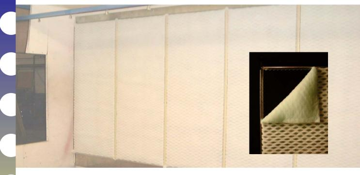
Paint Pockets® Zipper™, Zip-It™, and other Accessories are designed specifically for use with Paint Pockets arrestors. The Zipper Mounting system Eliminates Spray Booth exhaust filter mounting worries while at the same time allowing you to get maximum utilization out of your Paint Pockets Overspray Arrestors:
